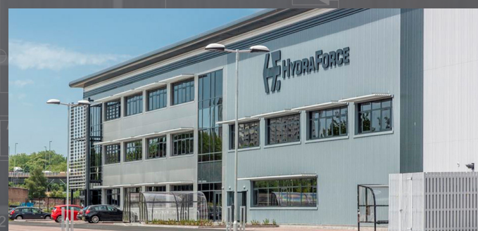
European Headquarters, Engineering and Manufacturing facility in Birmingham, England
