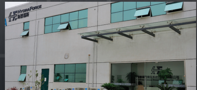
Asian/Pacific headquarters, precision machining and manifold assembly facility in Changzhou, China, near Shanghai.
