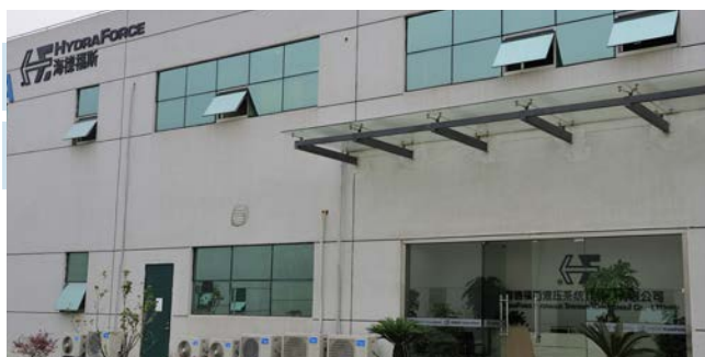
ASIAN/PACIFIC HEADQUARTERS, PRECISION MACHINING AND MANIFOLD ASSEMBLY FACILITY IN CHANGZHOU, CHINA, NEAR SHANGHAI.
