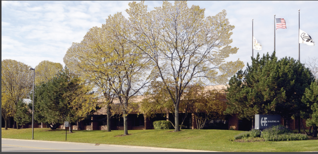
Main headquarters, engineering and manufacturing facility in Lincolnshire Illinois, just north of Chicago.
