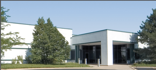
Precision machining facility in Lincolnshire, Illinois.
