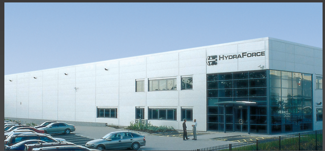
European headquarters, engineering and manufacturing facility in Birmingham, England.
